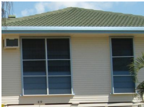
Figure SC6.2.3.17 Illustrates an example of a full height window, acceptable in 1960’s Defence Housing Precinct only
